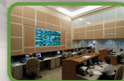
Traffic Management/Operations Center
